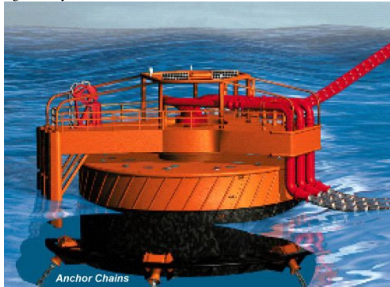
Figure 5 Typical buoy layout with offloading lines and anchors
